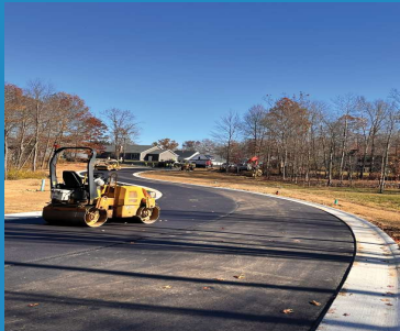
Treemont Estates No. 3 Paving & Curb Canton Township
