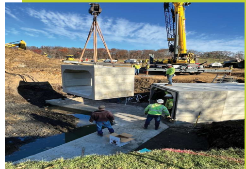
The Glens of Jackson No. 1 & 2 Assembling a Box Culvert Jackson Township
