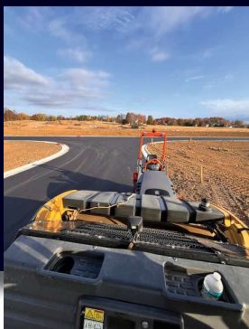
Frank Farms No. 1 & 2 Riding the Compaction Roller Jackson Township
